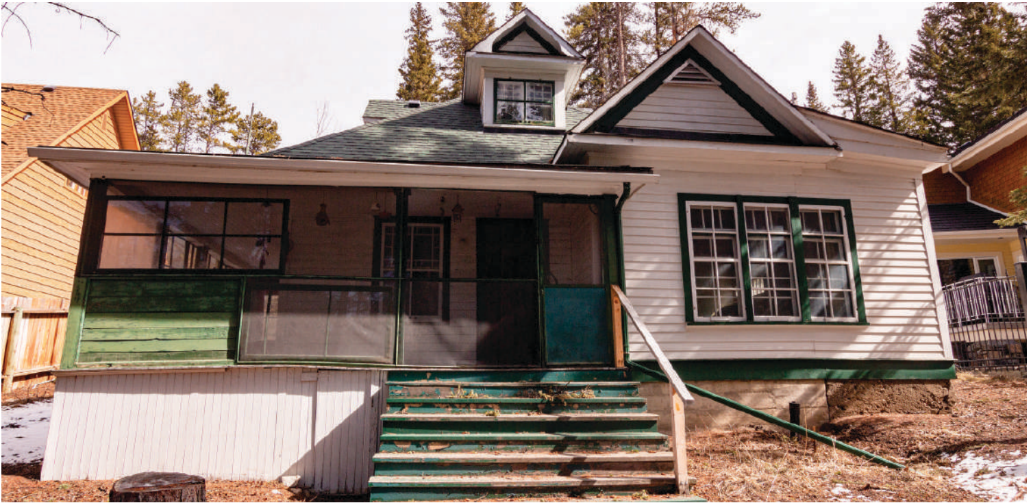
Plans are underway to restore the historic 1908 Rutherford House in Banff – the former summer cottage of Alberta’s first premier Alexander Rutherford.
