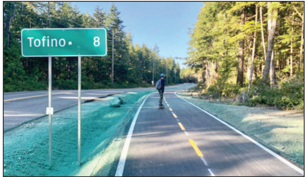
The District of Tofino is preparing to build an extension to its Multi-Use Path . (DoT file photo)
