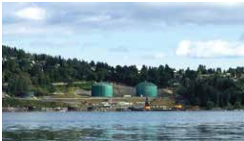
Trans Mountain pipeline’s Westridge Marine Terminal on the B.C. coast, pictured July 2019, is being upgraded as part of the expansion project. Wikimedia Commons photograph courtesy of Codex.
