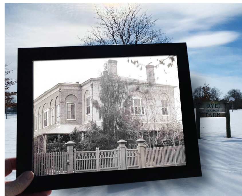
This building once stood on what is now Rye Park. It was the courthouse and jail for NOTL in the 1800s and the scene of the so-called Moseby riot. Solomon Moseby escaped slavery in Kentucky in 1837, travelling north on his owners' horse. His former owner followed him to Niagara and demanded his extradition. Moseby was arrested and jailed. Both Black and white residents petitioned the lieutenant-governor to refuse the extradition, but the order was signed. Two hundred or more Black people, many of them women, gathered to protest peacefully at the jail. But when a carriage carrying Moseby appeared, two protesters tried to stop it, and shots were fired by order of the sheriff. Moseby escaped in the chaos. The two men who intervened died and two others were severely injured.
