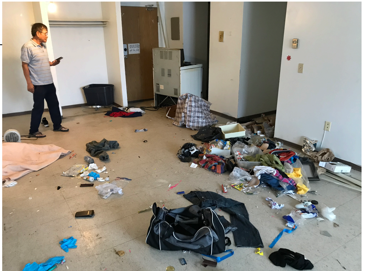
Hien Tran, president of the Free Vietnamese Association of Manitoba, surveys garbage left in a suite. The two-bedroom suite was one of six with damage caused by squatters, including broken plumbing fixtures and walls marred by holes and graffiti. Photo Sean Ledwich
