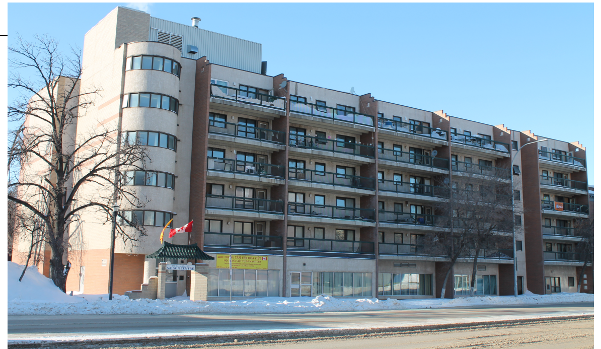
Owners of the Saigon Centre on Balmoral Street accuse Manitoba Housing of leaving behind a legacy of disrepair. Photo Sean Ledwich
