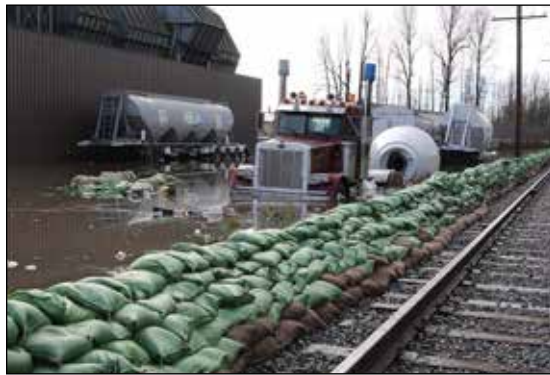
Sandbags along the railroad tracks in Huntingdon Village kept the floodwaters from reaching homes. (Wikki Hopes/Abbotsford News)
