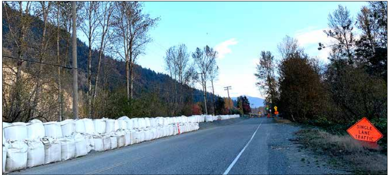
Gabions are still in place along North Parallel Road in Abbotsford leading to Barrowtown. (Jessica Peters/Abbotsford News)
