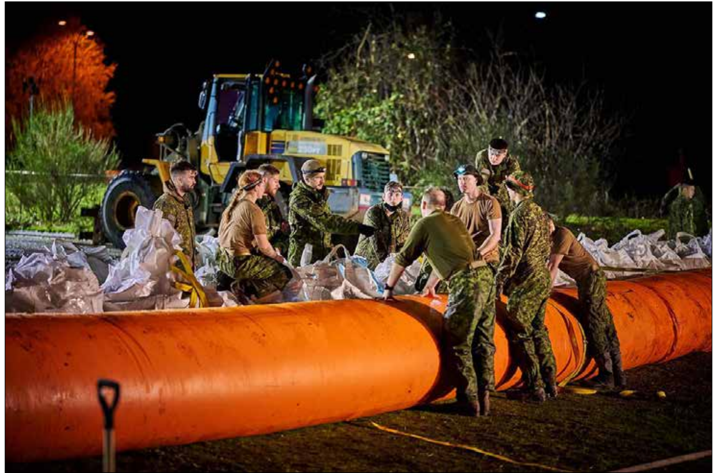
Military crews helped place a Tiger Dam across Highway 1 near Cole Road in Abbotsford on Nov. 28, 2021. (Abbotsford Police Department photo)
